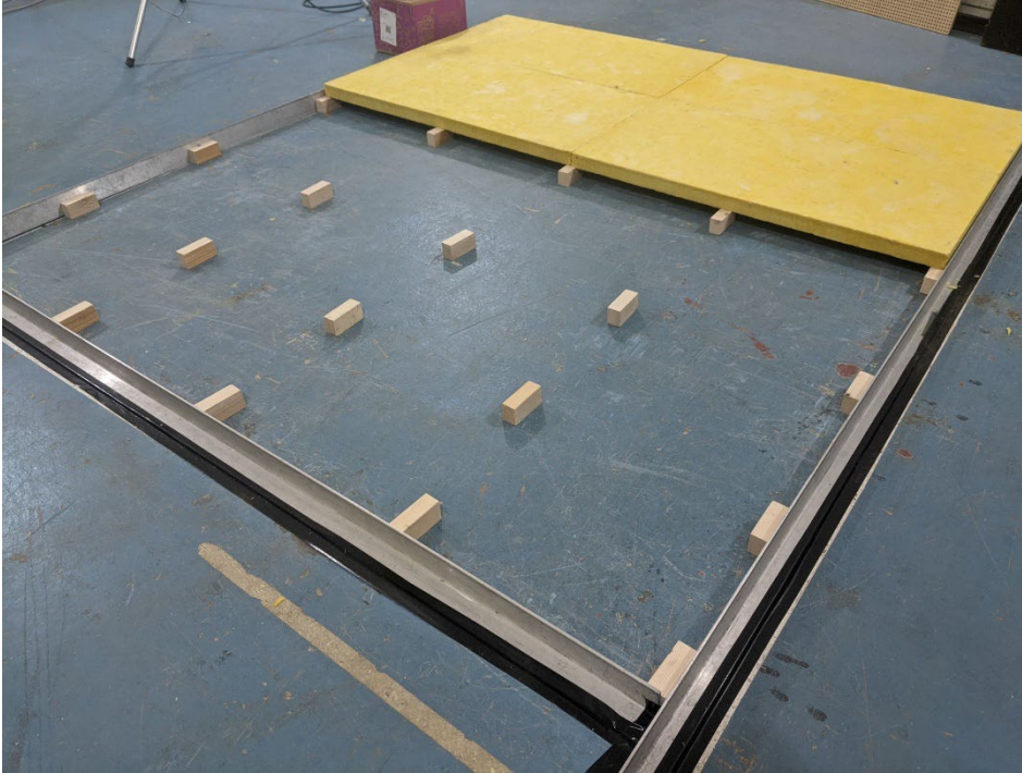
Figure 3 – Base layer of fiberglass partially installed over spacers
